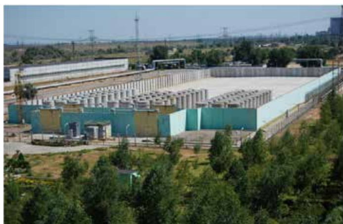
Dry Storage Facility (DSFSF) at the Zaporizhzhia site with concrete dry storage casks
